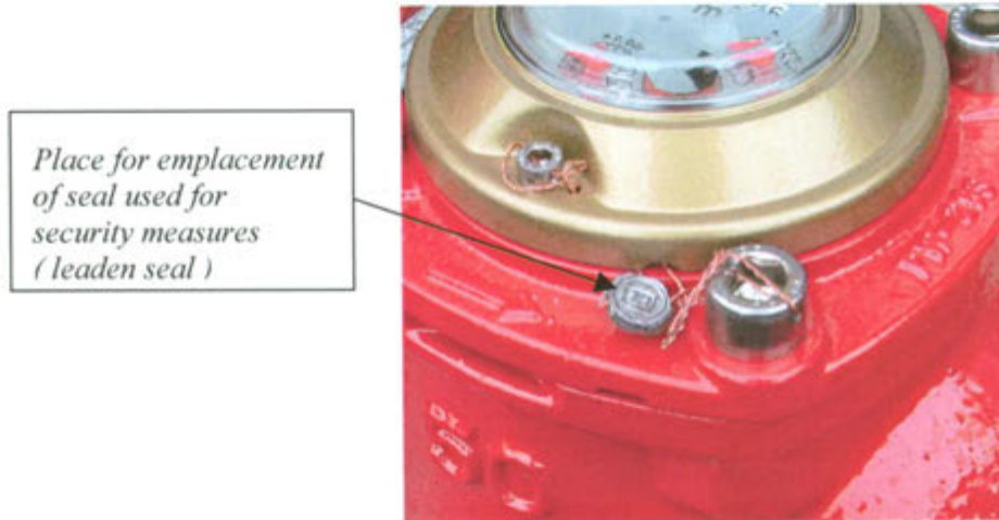
Picture No.2 Emplacement of the seal for security measures
